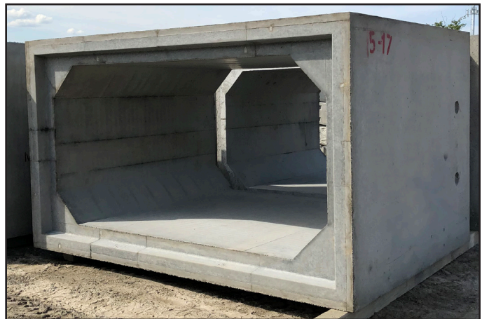
Finished Box Culvert
