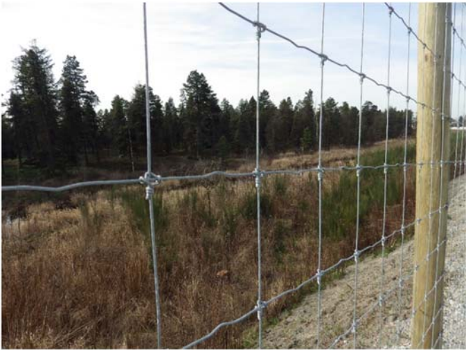
Game fence installed on a ranch
