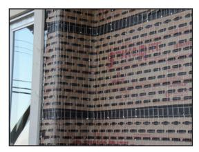
Stucco-Rite® is designed with an open lug, reducing the need to add costly installation time for the installer to manually eliminate an unwanted cold joint.
